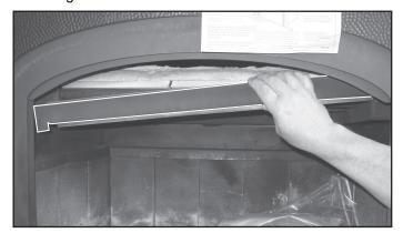
Figure 4.5 Removing Baffle Protection Channel
