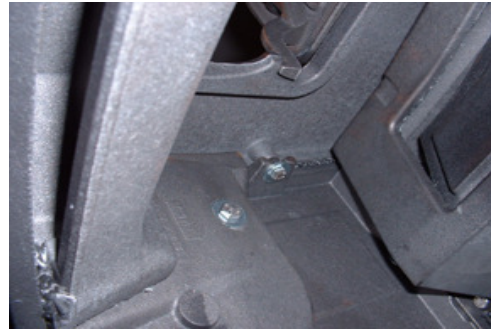
FIG. 2 Interior Top Attachment Hex Head Bolt
