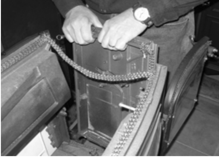
FIG. 18 Lift Right Side From the Stove
