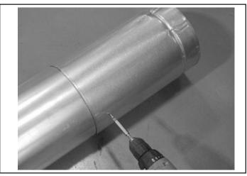
Figure 3.5 - Screws into Slip Section
