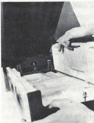
Loosen nuts and washer at bottom of each side tile section, and remove nuts and washer at top. Insert bottom bolt in slot at base of firechamber.
