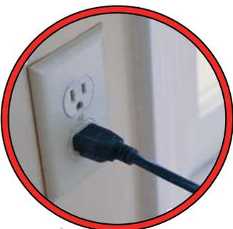
If the Optional Fan Kit is installed, connect this unit to a properly grounded, 110-volt electrical outlet. Do not route the power cord in front of, or under, the stove.
