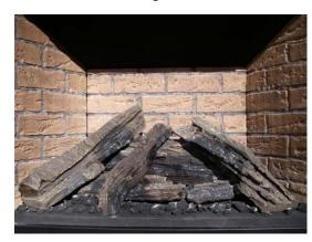
Step 5: Place right log on rear log and front of burner as shown.
