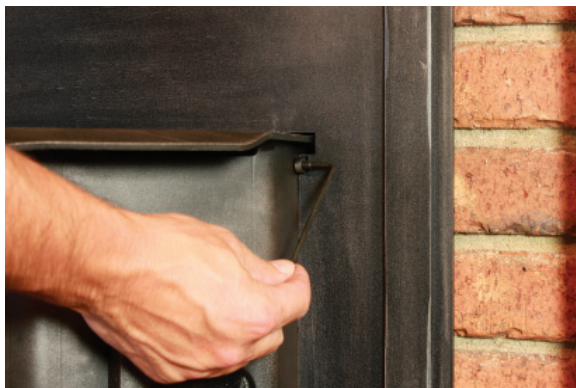
FIREPLACE INSERT SURROUND PRESSURE SCREWS
