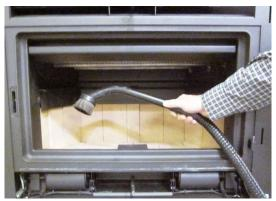
2. Carefully place the brush surface of the nozzle over the catalytic combustor openings and remove any ash or debris. Take care to prevent damage to the catalytic combustor (the surface is fragile).
