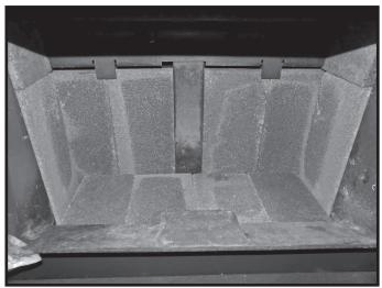
Figure 28: Firebrick placement complete.
