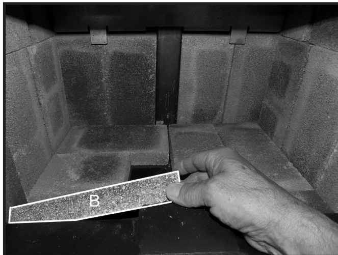
Figure 30: Final narrow brick in place.
