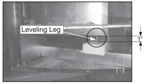
**Figure 13.2.** Ensure that the leveling leg is positioned over the  $2 \times 4$  before leveling the insert. Minimum 1" clearance.
