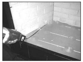
**Figure 12.3**. Using a saws-all, cut out the floor.
